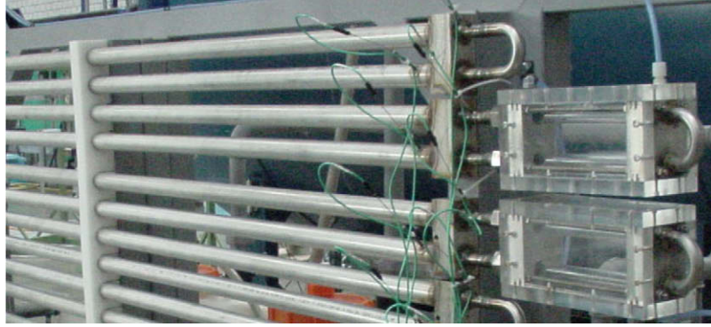
Fig. 2. Evaporator (before thermal insulation) with sight glasses.
